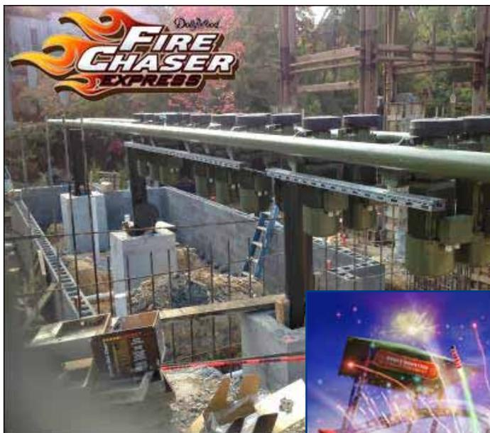
After conferring with SpecChem on the parameter of their job, Dollywood Construction Group, of Pigeon Gorge, TN selected SC Precision Grout to form baseplates at the bottom of Dollywood's newest roller coaster. Dollywood Construction Group needed a grout with excellent flowability and high early strength gain to ensure the roller coaster had maximum stability to endure the incredible "G force" of the roller coaster.
