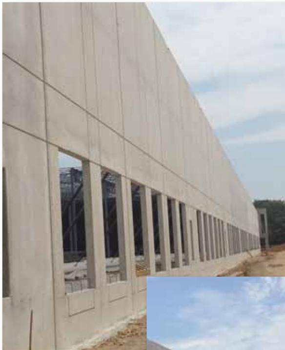
MK Concrete Construction of Frederick, MD recently completed tilt-up operations on the Landover Logistics project using SpecTilt WB cure & bondbreaker. Resulting panels were smooth and tight, exceeding expectations.
