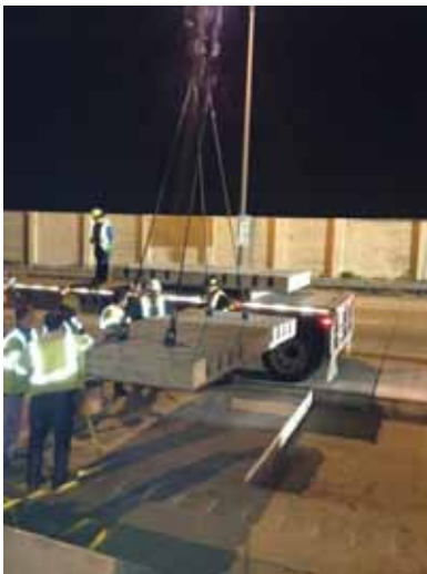
Precast Slab Placement
